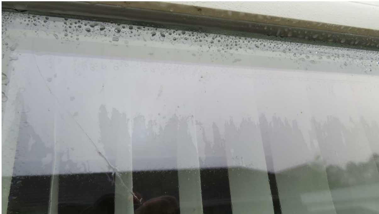
Droplets on the glass caused by silicone joint ...Gouttelettes causées par les joints de silicone
